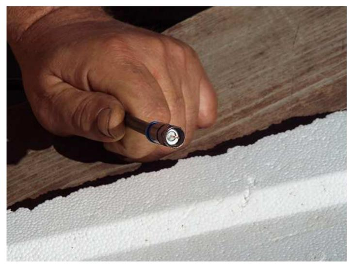
Carefully make sure that no small wires can cause possible shorting and that the center insulator is flush with the connector bottom as shown.
