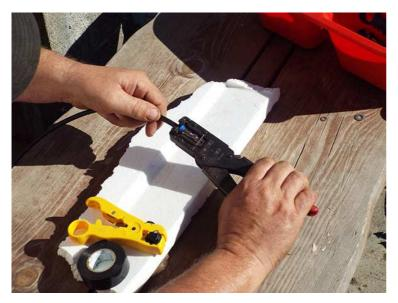
Begin squeezing the handle to press the blue sleeve into the connector shell.
